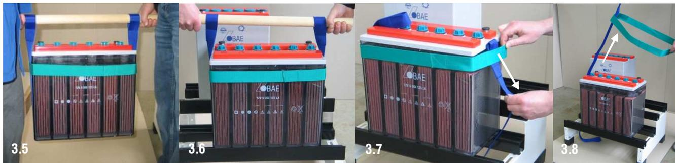
3.5 Insert the wooden bar through the two clips and carry the block by two persons.
